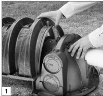
1 Place first chamber onto end cap.
