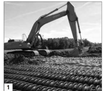
1 Ladle the fill.
